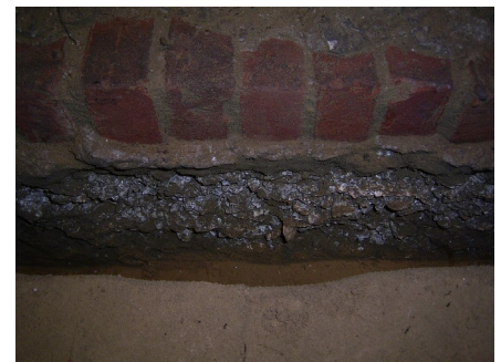
Figure II-113. Close-up of north foundation wall and oyster shell layer in builder's trench.
