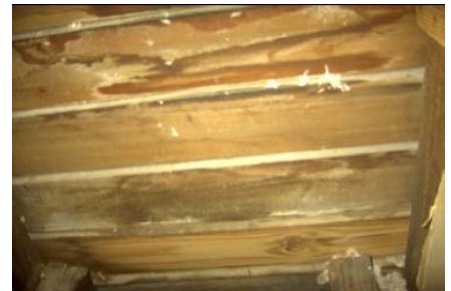
Figure II-89. Interior surface of wood clapboard siding.
