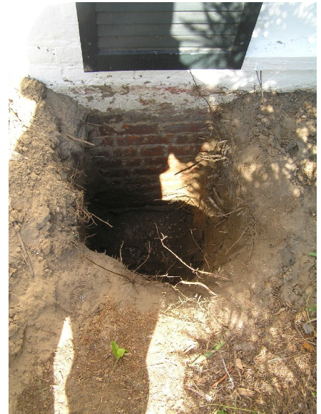
Figure II-6. LAS Test Unit excavated below column bearing point. Investigation revealed continuous foundation wall below grade. Coursing matched adjacent walls precisely. No evidence of masonry footing was present.
