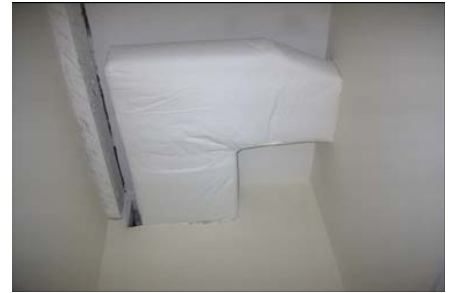
Figure II-85. Exposed duct, first floor restroom.
