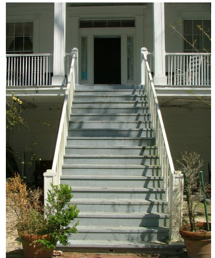
Figure II-19. Detail view of rear stair and porch details.
