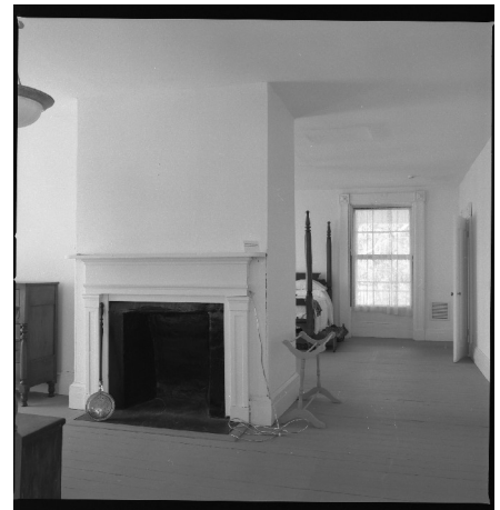
Figure II-51. Second Floor Bedroom.
