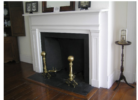
Figure II-78. Wood fireplace mantel located in first floor Dining Room.
