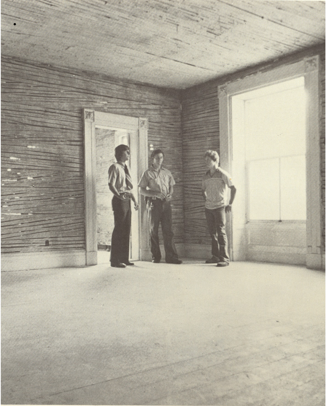
Figure I-14. Title X Program team members, School Counselor Bob Hemminger, Vocational Teacher Carlos Jones and student Richard Bryson in second floor bedroom after removal of wall and ceiling plaster.
