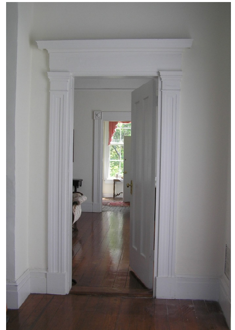
Figure II-50. First Floor Door Casing.
