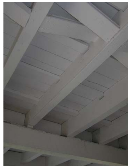
Figure II-31. Notching of Ceiling Joists to Accommodate Sleepers.
