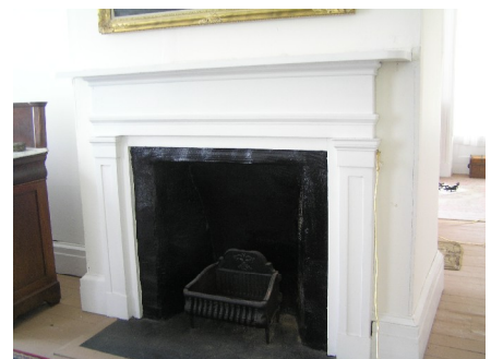
Figure II-79. Wood fireplace mantel located in second floor bedroom.
