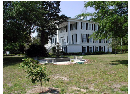
Figure II-105. View of Property Looking Southwest.
