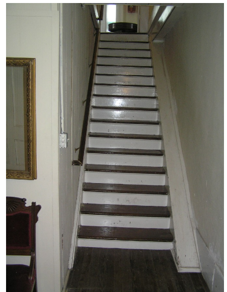
Figure II-40. View of Stair B03.
