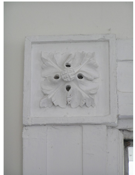
Figure II-17. Detail view of corner block at Second Floor door casing.
