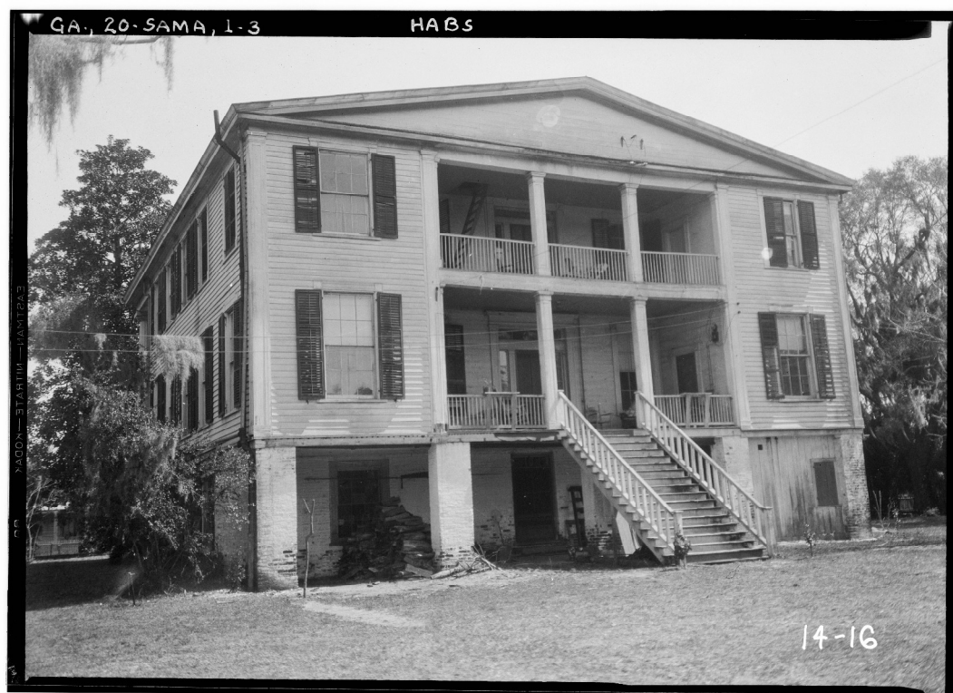
Figure I-12. Rear Elevation of Orange Hall in 1934. HABS Photograph.
