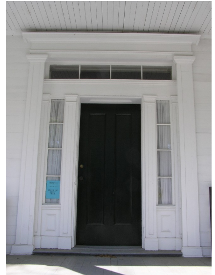
Figure II-16. Rear entry door at First Floor Level.
