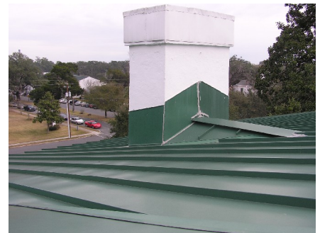
Figure II-21. Detail of existing standing seam metal roof.
