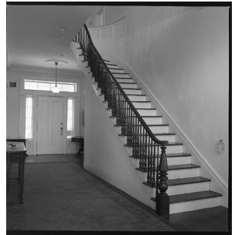
Figure II-48. View of First Floor Central Hallway.
