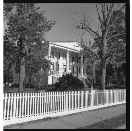
Figure II-1. View of Orange Hall from Osborne Street
