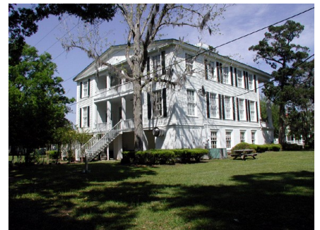
Figure II-108. View of Property Looking Northeast.
