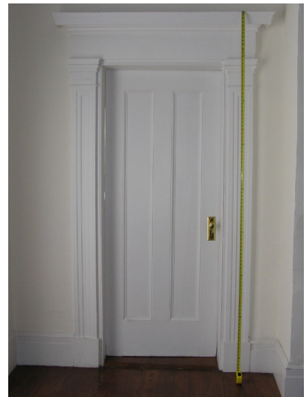
Figure II-52. Typical Interior Door at First Floor.
