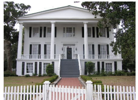
Figure II-9. Image showing step in wood trim at transition between masonry foundation and wood clapboard siding.
