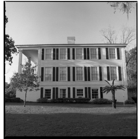
Figure II-5. North elevation of Orange Hall showing masonry foundation wall.
