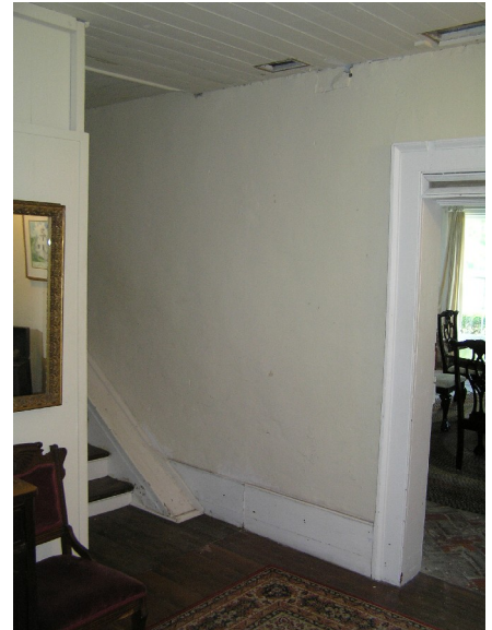
Figure II-38. View of Hall B01 looking toward stair to first floor.
