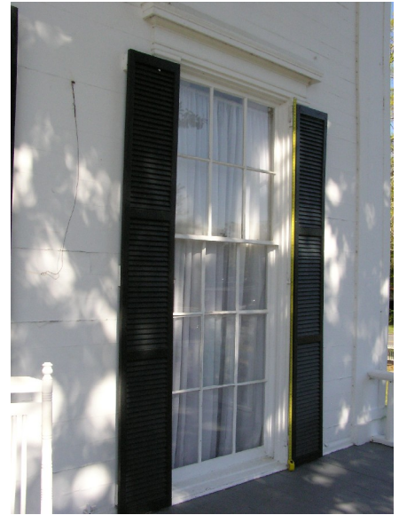
Figure II-13. Typical six-over-nine, window located at the First Floor, East Elevation.
