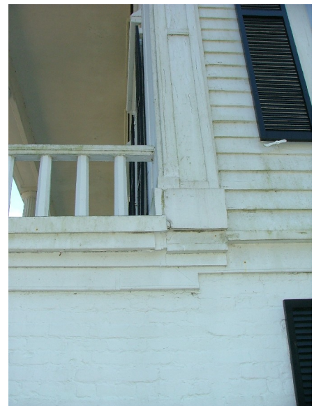
Figure II-8. Image showing step in wood trim at transition between masonry foundation and wood clapboard siding.
