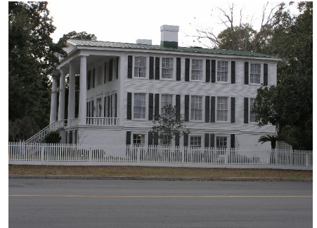
Figure II-20. North elevation of Orange Hall. Note roofing material is barely evident due to low slope.
