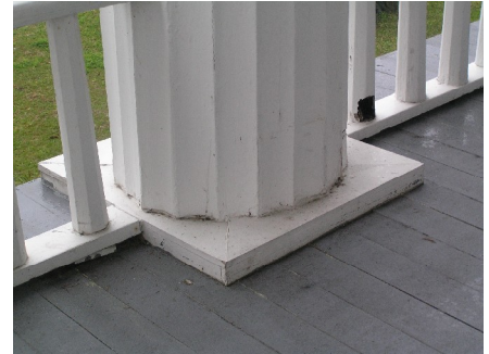
Figure II-11. Base of column showing added base element. Originally, no base was present, with the column shaft terminating directly into the porch floor.
