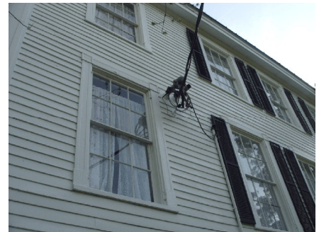
Figure II-90. Weatherhead on side of building.
