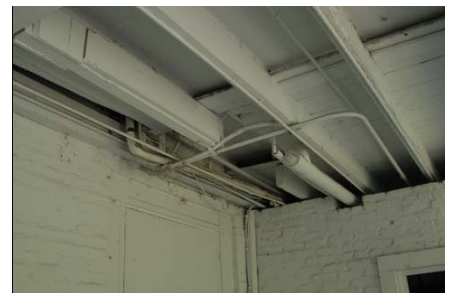
Figure II-28. Structural Members that have been Cut at Rear Porch.
