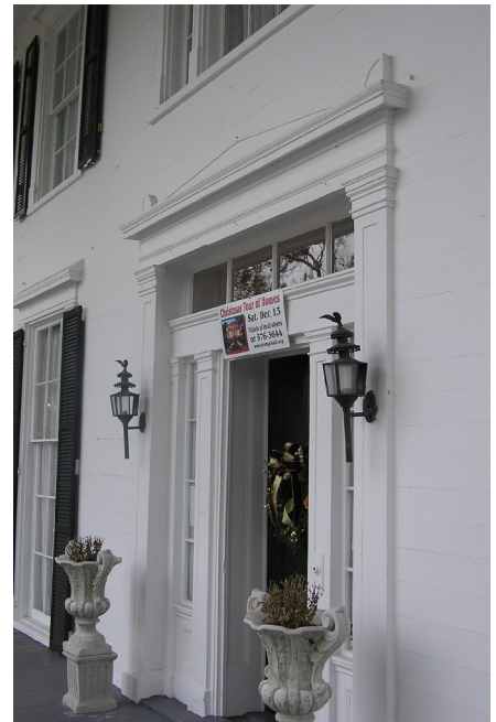
Figure II-15. Main entrance, Orange Hall.
